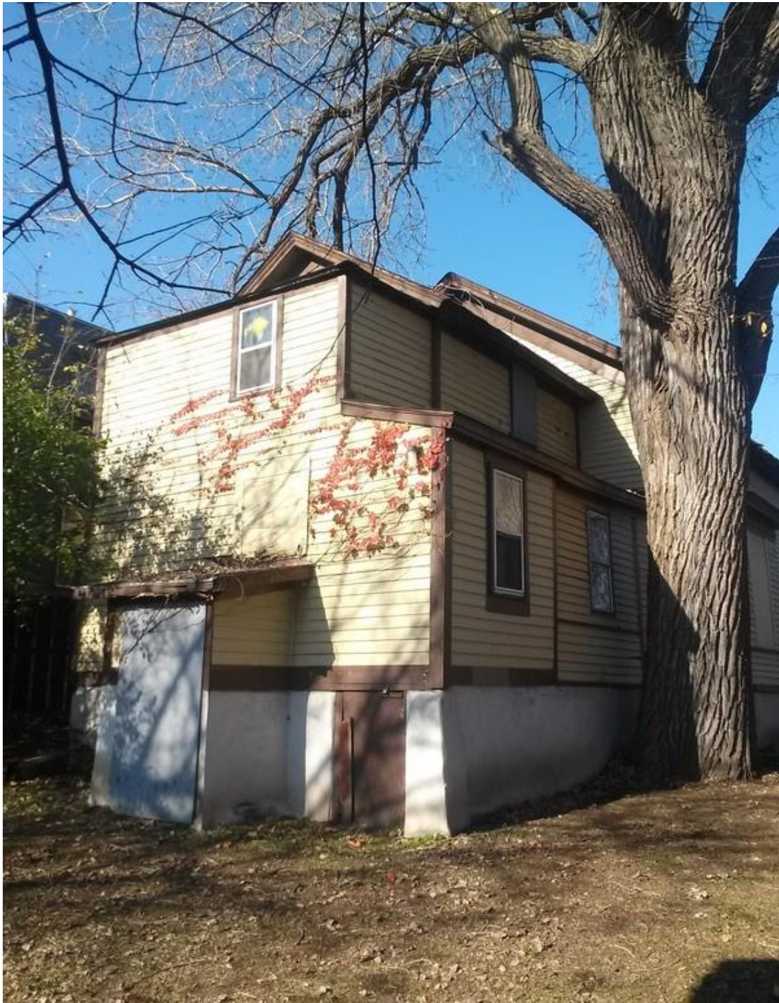
656 Bush Avenue back of house with multiple additions 2015
